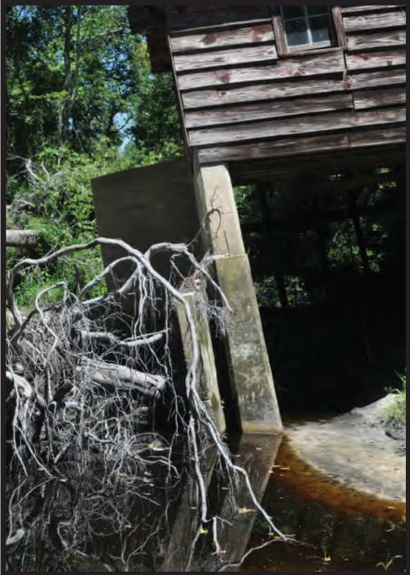
Figure 15. Detail of West Foundation Wall
